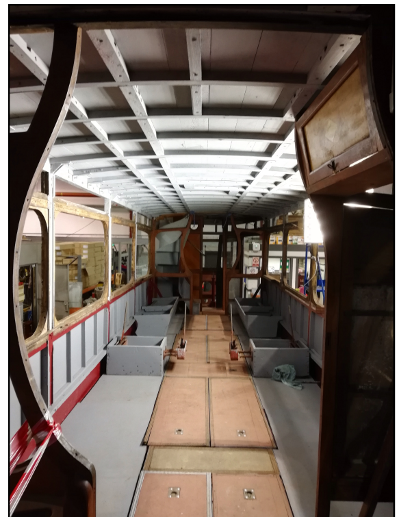
Work is now concentrating on the inside of 1245
