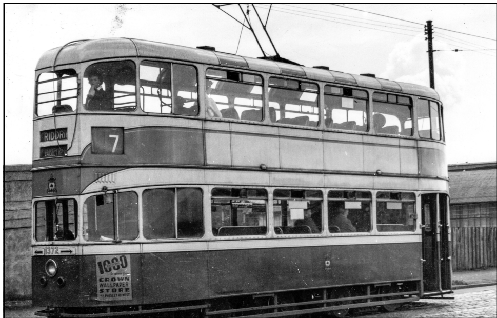
Cunarder 1372 at Bellahouston terminus in Jura Street on 7th August 1954. The upper deck front window is still in original condition as a full width drop pane, soon to be modified with the small opening central window to access the bow rope. (photo courtesy RJS Wiseman)
